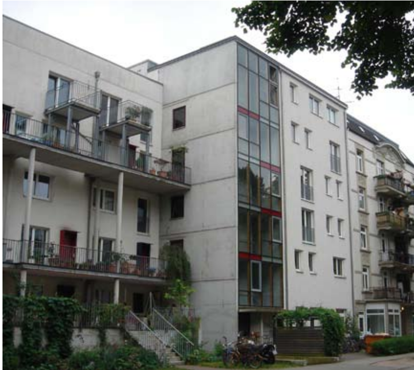
Passive house in Hamburg, Telemannstraße
